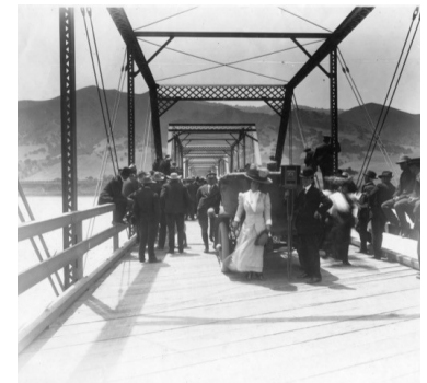
Opening of San Ardo Bridge April 1908
